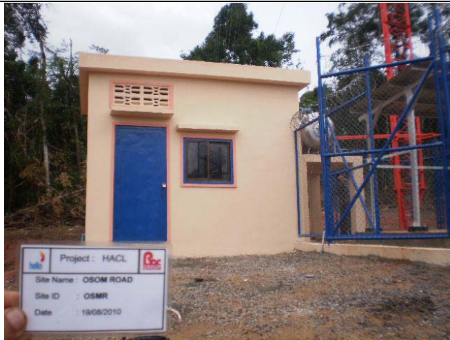
Guard Room External Front View
