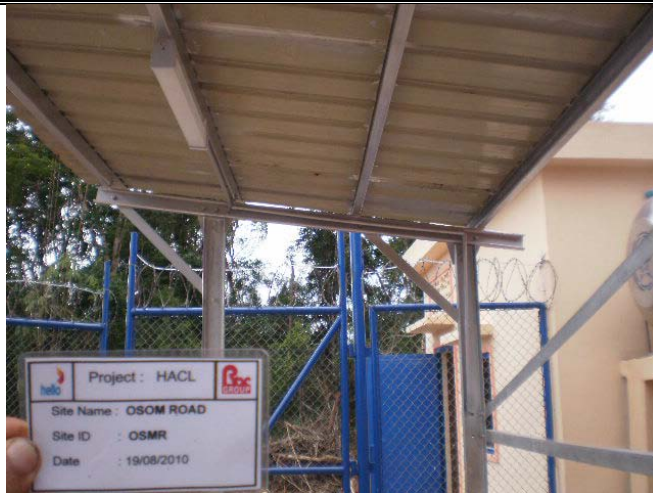
Shelter Right Side View
