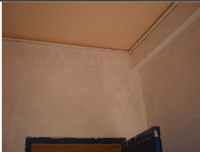
Guard Room Ceiling
