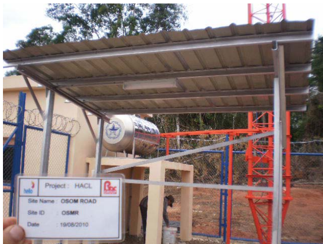
Shelter Front View
