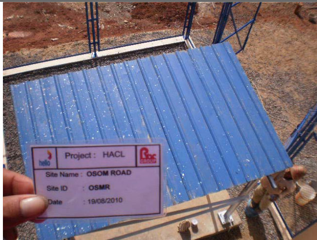
Roof ( Taken from Tower)
