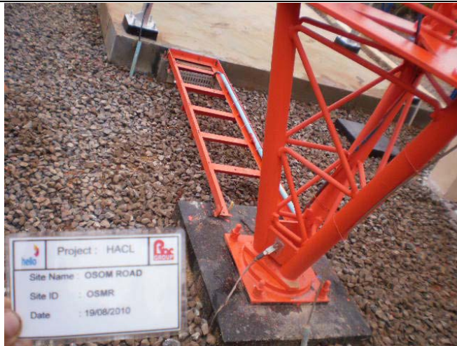
Grounding Connect to Tower ladder
