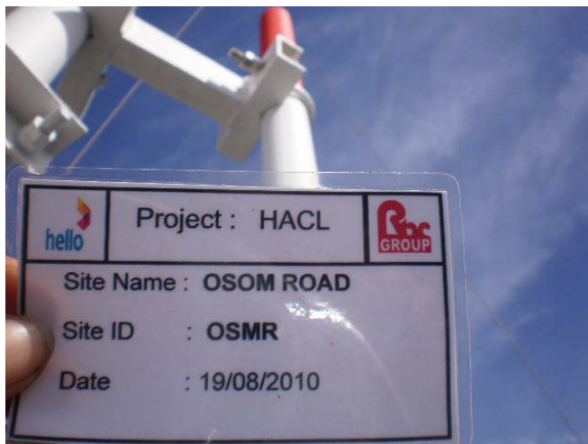
Antenna mounting Installation ( right)
