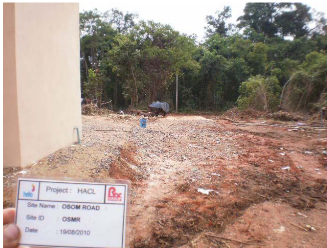
Guard Room Right View
