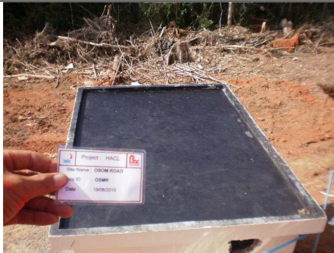
Guard Room Roof ( Taken from Tower)
