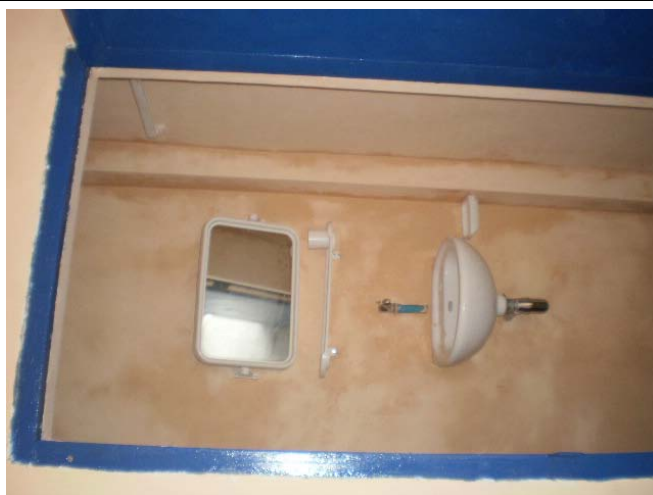
Sewage System & Septic Tank
