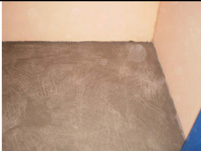
Guard Room Interior wall View
