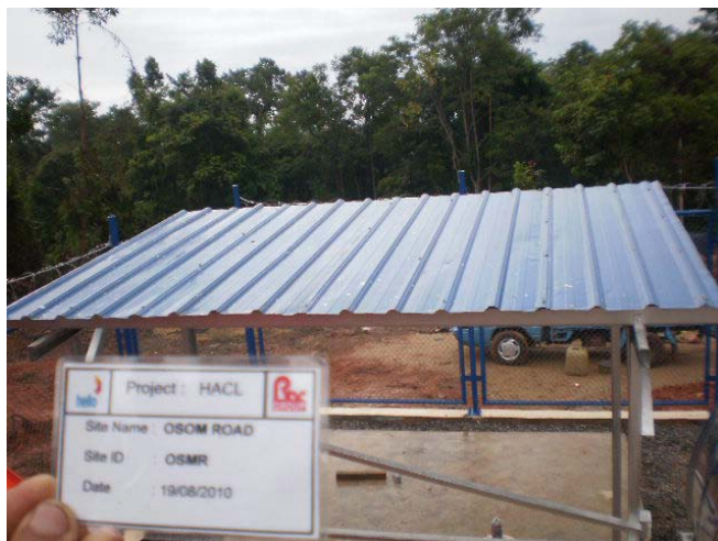
Shelter Rear View
